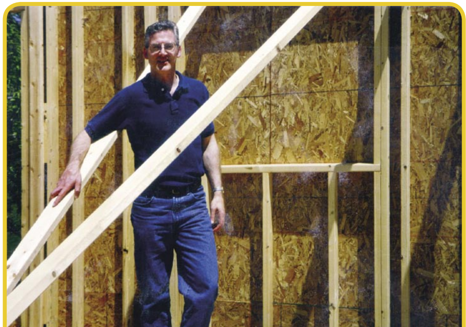
If you build it... Paul visits the Mettler Center construction site in the spring of 1997.
